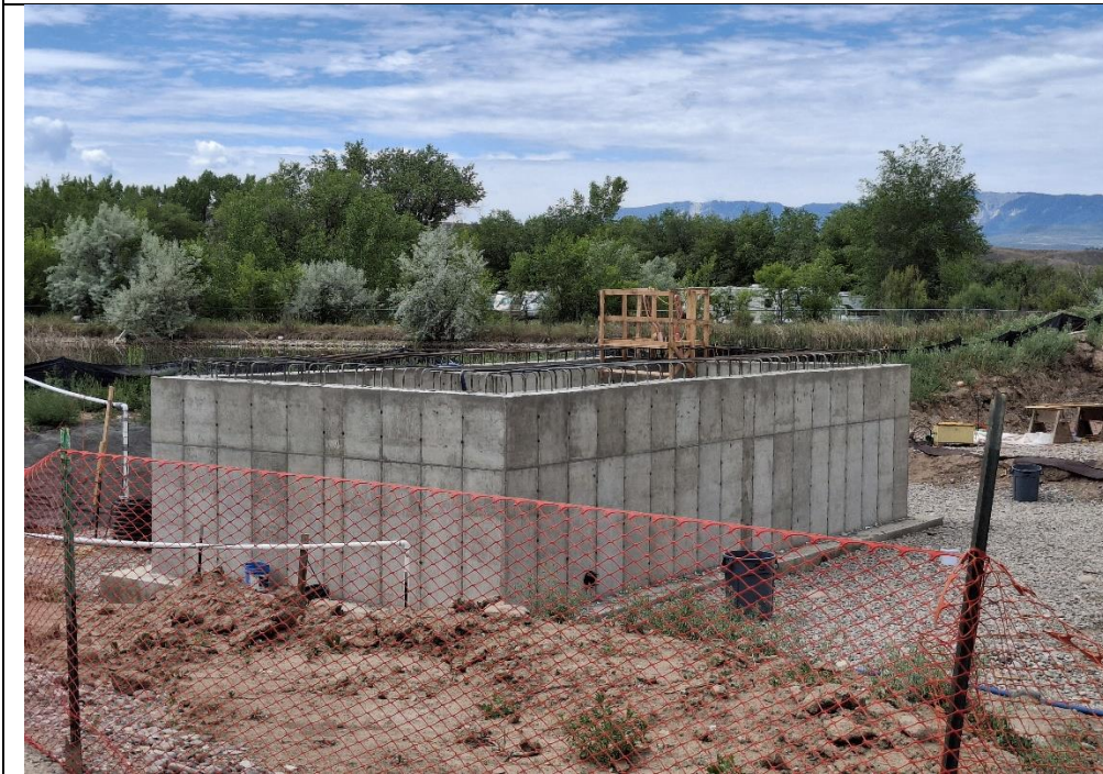
Backwash Tank Concrete
