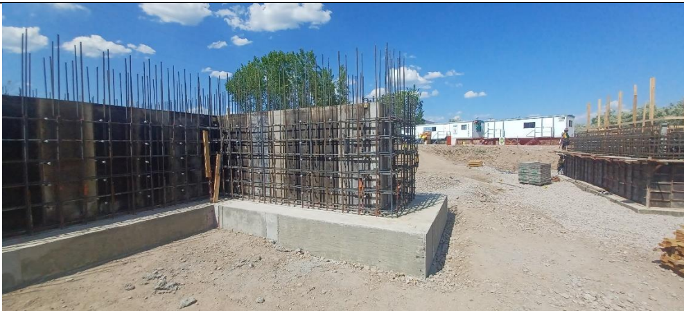
Chemical Trench Wall Rebar & Formwork
