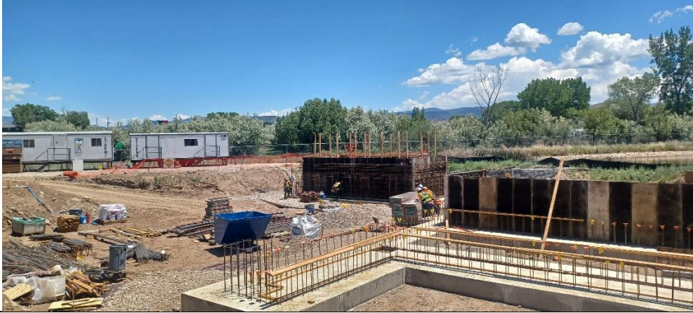
Backwash Tank Wall Forms & Rebar
