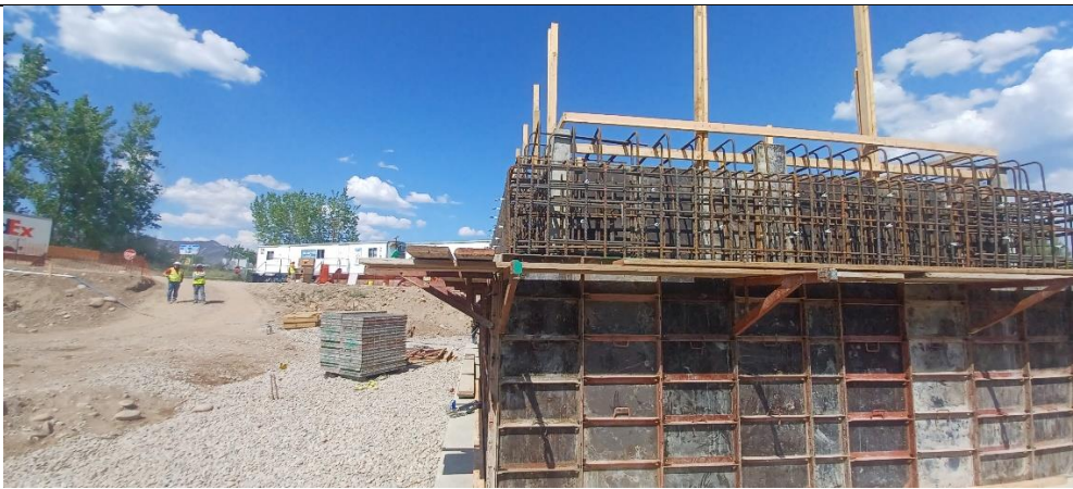
Backwash Tank Wall Forms & Rebar
